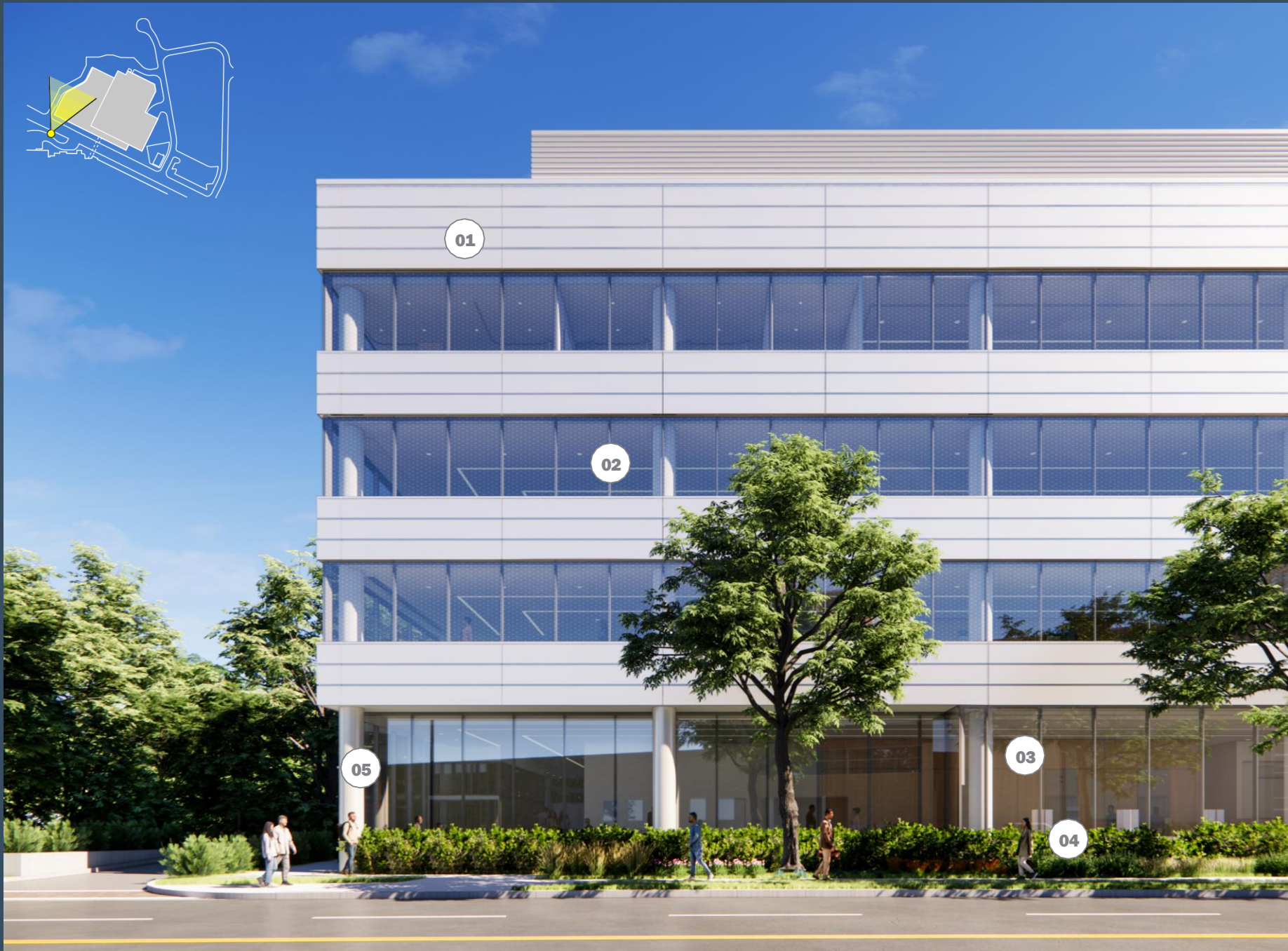
02 REFLECTIVE VISION GLASS - 1/8" DOT S, 2" INLINE BIRD FRIT
