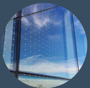
VISION- SEMI REFLECTIVE WITH 1/8" DOTS, 2" INLINE BIRD FRIT
