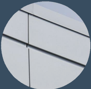
01 PREFINISHED INSULATED METAL PANEL – SILVERSMITH METALLIC FINISH
