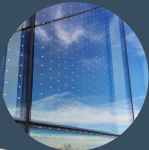
02 REFLECTIVE VISION GLASS - 1/8" DOT S, 2" INLINE BIRD FRIT
