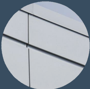
01 PREFINISHED INSULATED METAL PANEL – SILVERSMITH METALLIC FINISH
