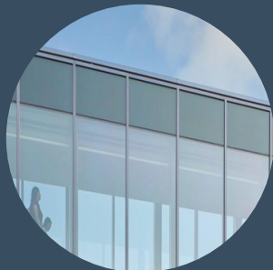
03 SPANDREL GLASS - 1/8" DOT S, 2" INLINE BIRD FRIT
