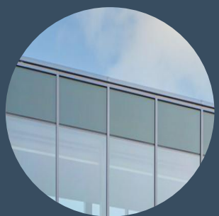
SPANDREL- CLEAR WITH 1/8" DOTS, 2" INLINE BIRD FRIT
