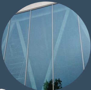
02 CLEAR VISION GLASS - 1/8" DOT S, 2" INLINE BIRD FRIT
